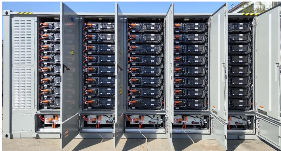
Figure 3 EnerC liquid-cooling energy storage container ---outside & inside overview
